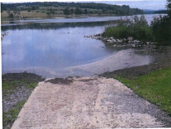
Photo 3: Existing concrete boat slip on Lough Gill
