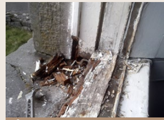
A window cill before repair works
