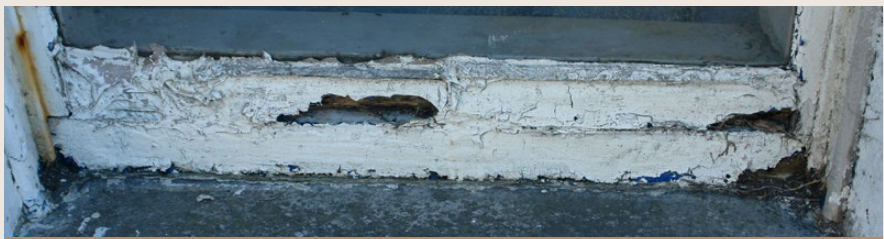
A window cill showing signs of rot and requiring attention
