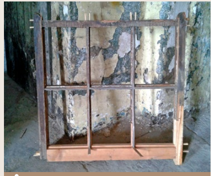
New timber has been used to replace rotten sections of this window sash.
