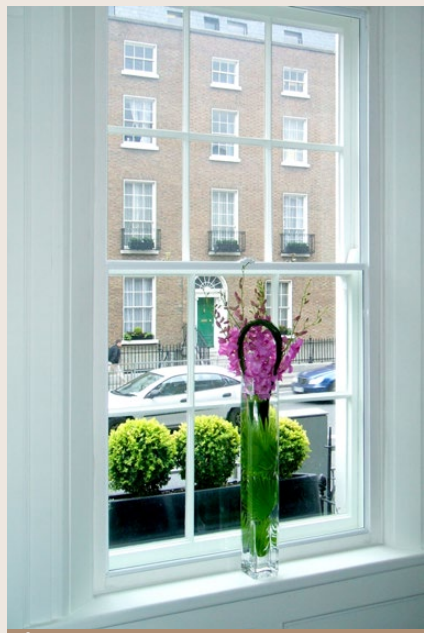
Successful unobtrusive secondary glazing on a Georgian building in Dublin
