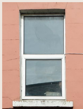
An inappropriate top-hung uPVC window
