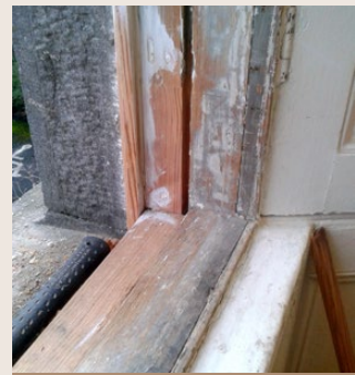
The same window cill after repair
