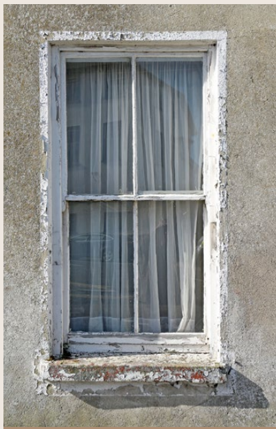
Deteriorating paint leaves timber vulnerable to decay
