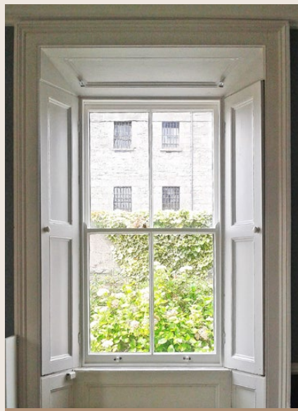
Inside a sash window at Governor's House, Sligo Gaol
