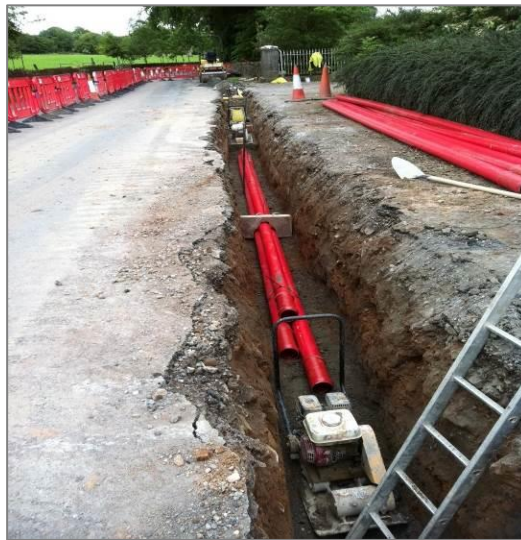
Figure 3 - Typical 38kV Underground Duct Installation (Single Circuit)
