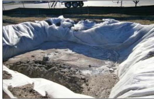
Plate 4-4 Concrete washout area
