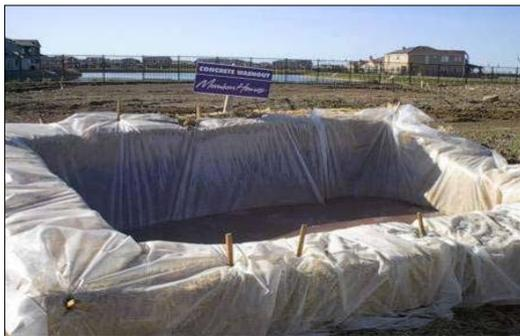
Plate 4-3 Concrete washout area
