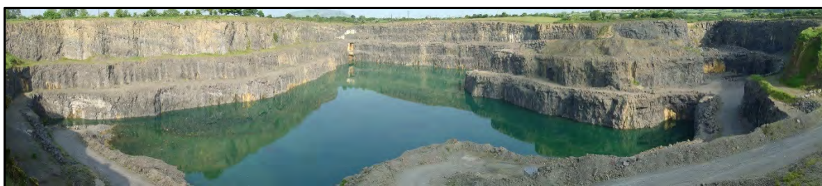
Plate 7-2: No pumping, quarry floor partially flooded (24/5/2018)
