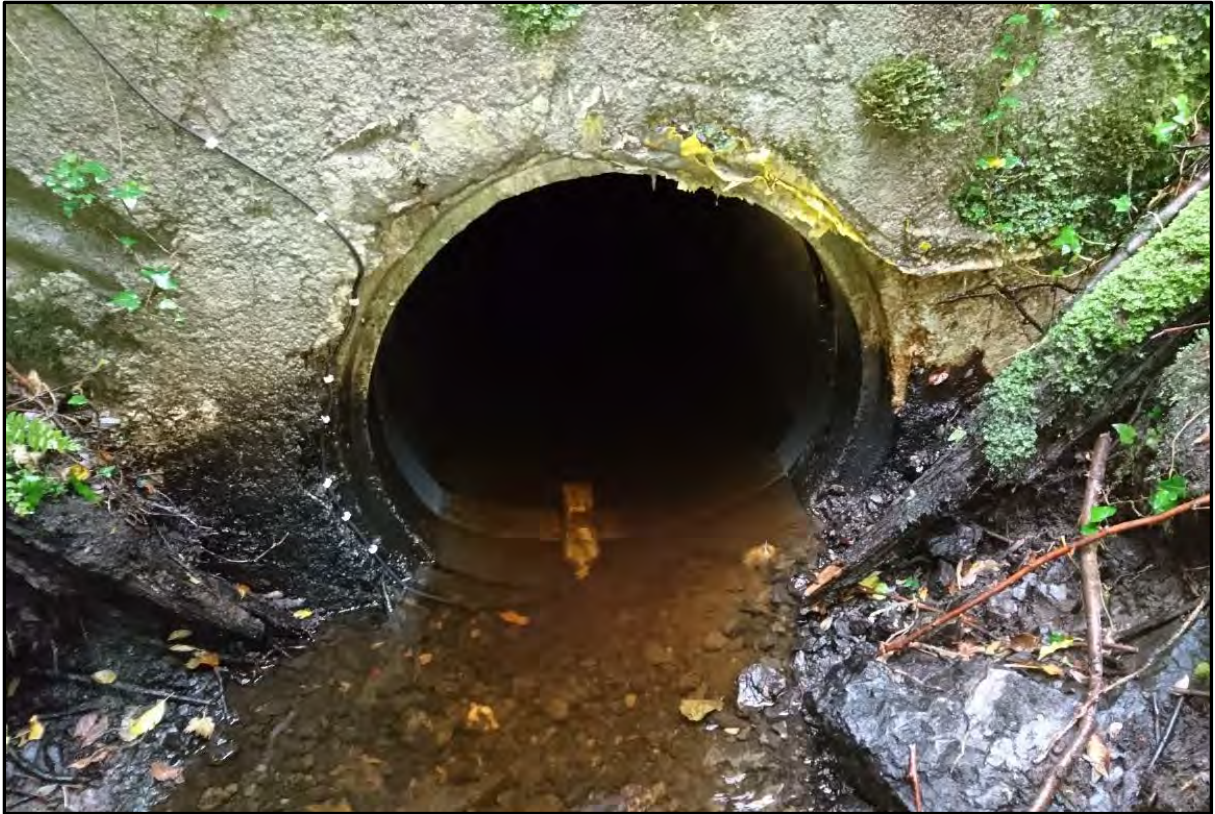
Photograph 3: Culvert 1 (downstream end) – Note Starflow flowmeter installed
