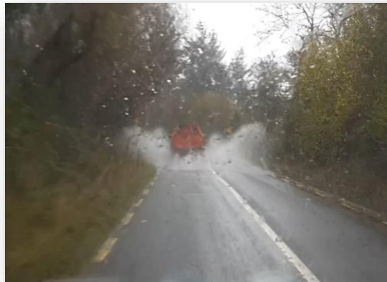
Figure 2-9: Existing N16 - Flooding/Aqua-plaining
