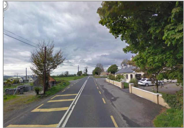
Figure 4.4 – On road access on N4 in Drumfin
