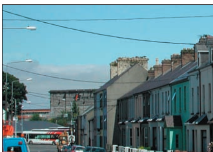
Negative visual impact of overhead cables
