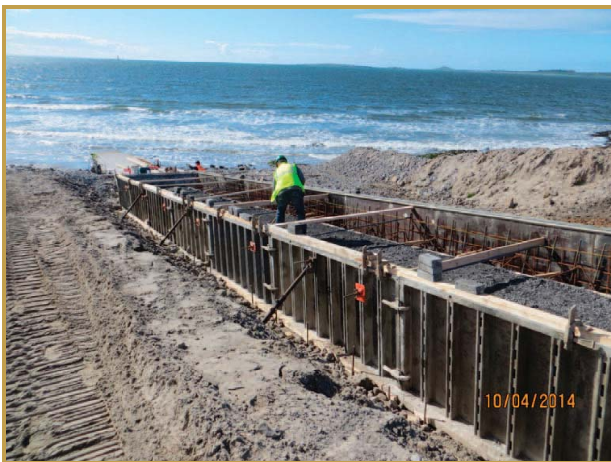
Replacement of failed beach access at rosses point first beach,
