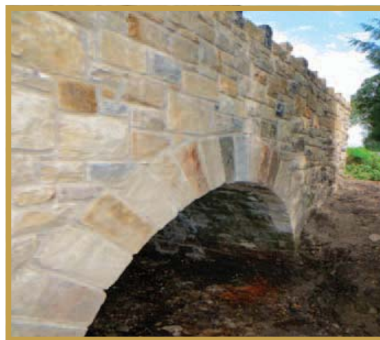
Aghoo Bridge – completed repairs
