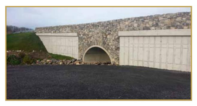
N59 Farranyharpy to Ballygreighan Scheme N59 works – new arch bridge and 2 retaining walls
