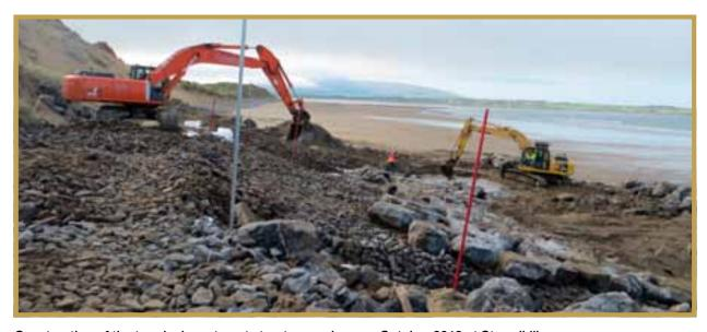
Construction of the terminal revetment structure under way, October 2013 at Strandhill.
