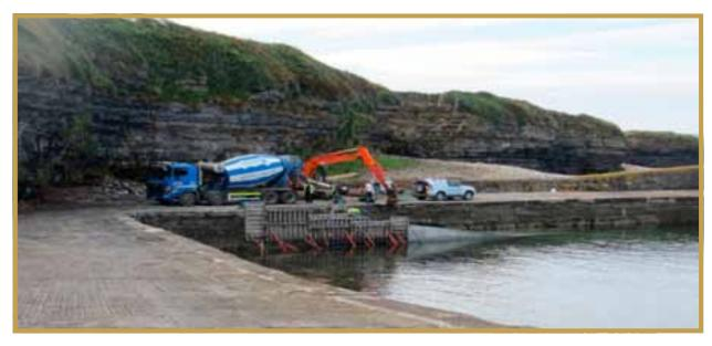
Slipway extension and regrading underway September 2013.
