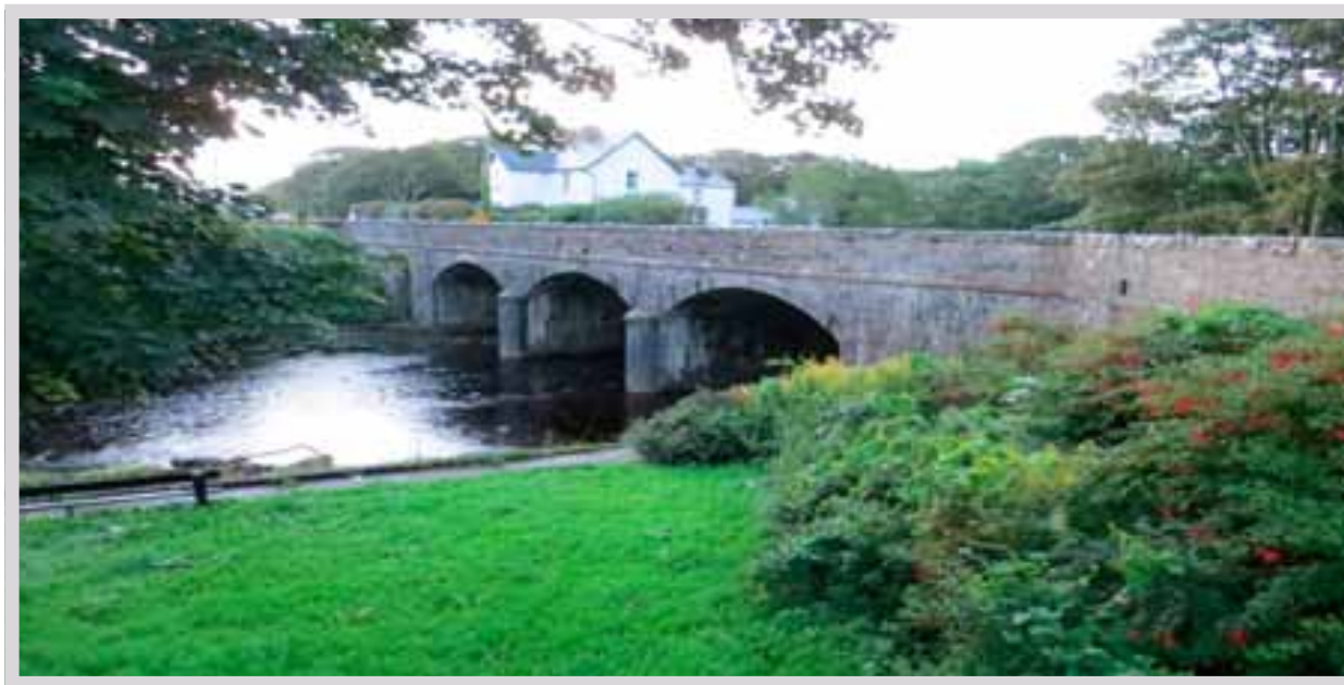
Easkey Bridge Restoration 2012. Parapets and spandrels repointed on this fine bridge, following vegetation removal. The bridge was designed and built by the county's first County Surveyor in 1850.
