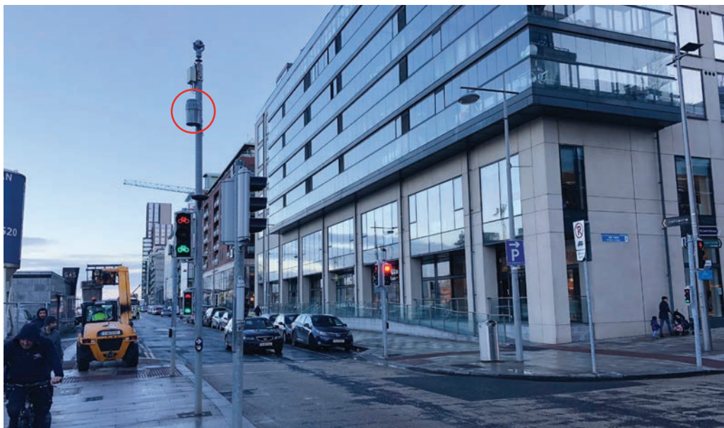
Example of deployed small cell.
