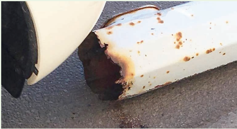
Example of compromised infrastructure
