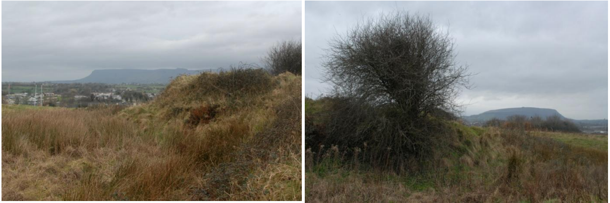
Fig.31: The main grassed entrance path to the west side of the fort shows animal erosion and damage from foot traffic in wet conditions within the defensive ditch.
