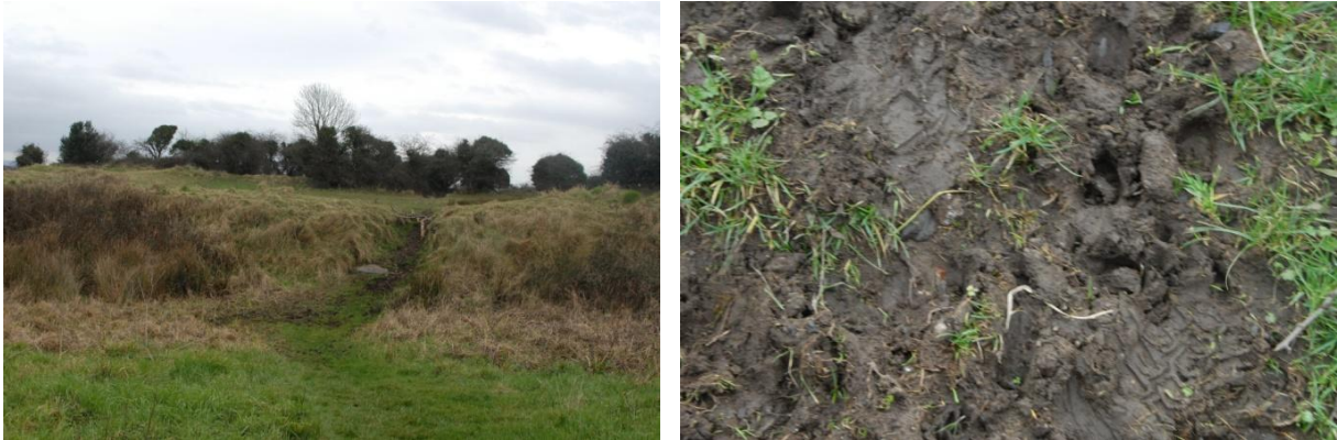
Fig.33: The main access onto the fort shows minor damage from human and animal traffic.
