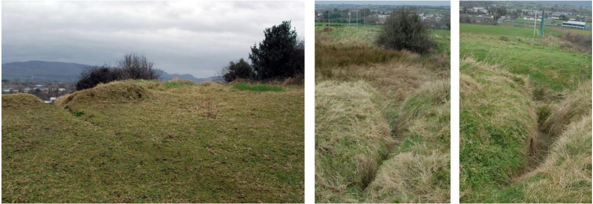
Above: Access routes on the north bank of the fort forming relatively deep cuts into the earthen banks.
