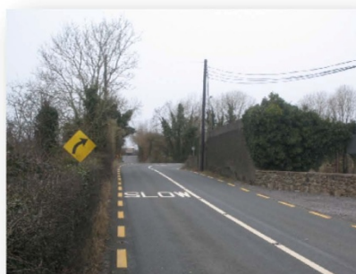
Figure 3-10: Junction with Drum Road (L-3406-0) which is a link to the N15 and is becoming increasingly busy
