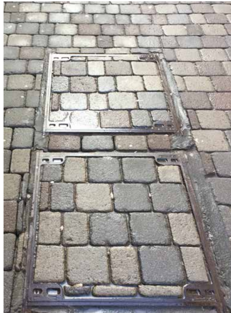
Paving infill cover with inconsistent gaps to paving
