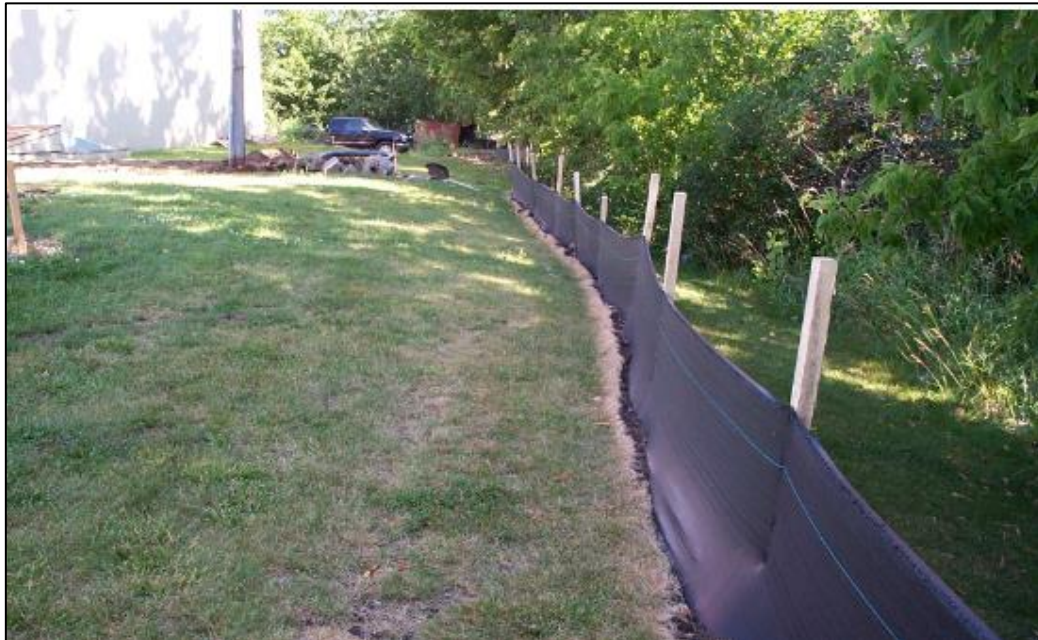
Figure 1.2.5: Example of silt fence in operation
