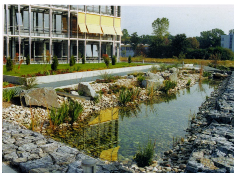
63 & 64: Examples of a stormwater retention facility incorporated into the landscaping plan of a business park. The example shown here is likely to require more maintenance than a simple ponds or reconstructed wetlands (see also photo 41), however such designs may be appropriate to the highly landscaped environs of a Business Technology Park.
