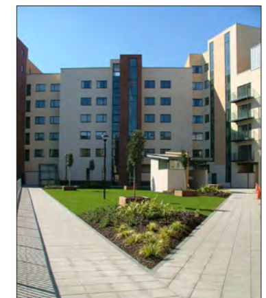
Mixed use courtyard development, North Cross, Dublin
