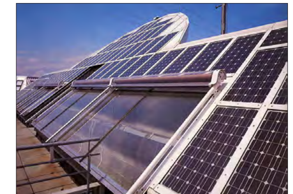
Example of Solar Panelling
