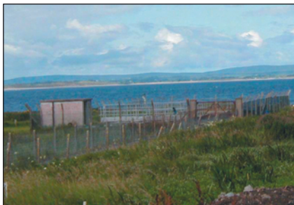
Wastewater treatment plant, Enniscrone
