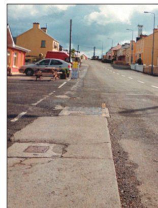
Existing footpath is poor in quality and is also hazardous in the manner it abruptly stops. The footpath should be continued and surface improved
