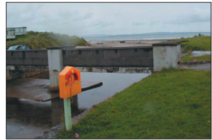
Bellawaddy Pedestrian Bridge, quite bleak and unattractive
