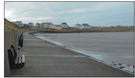
Promenade walk from the Hollow to the old seaweed bathhouse
