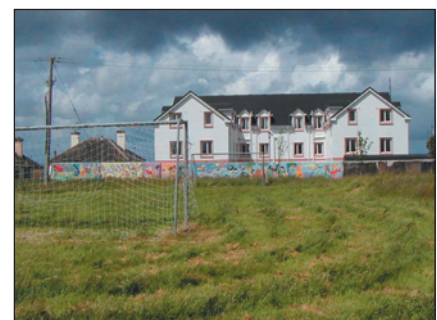
Open Space in county council housing estate, Enniscrone
