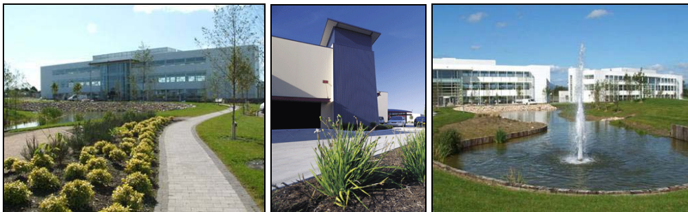
Landscaping and innovative layouts minimise the scale of large-scale industrial developments
