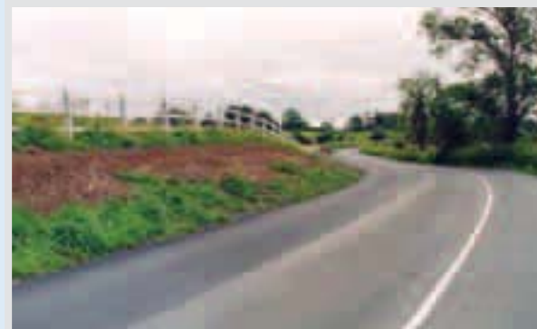
△ Alignment and resurfacing works on the R287 Crossboy
