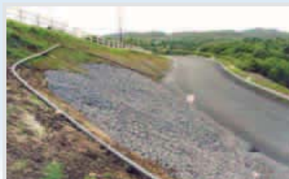
△ Alignment and resurfacing works on R290 Ballygawley-Collooney Road
