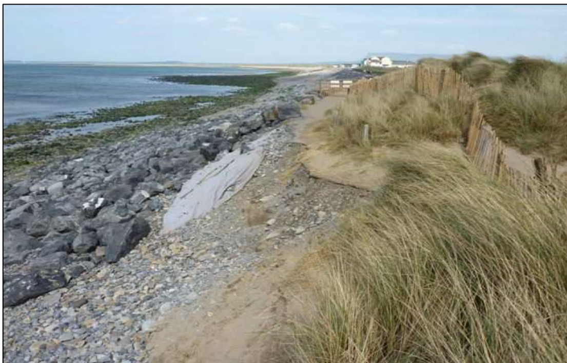
Figure 4.2: Damage to the transition zone and evidence of terminal erosion to the dune 5 th May 2011
