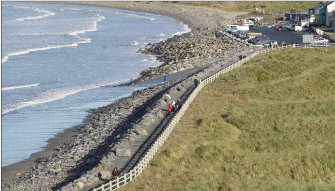
Figure 4.1: Rock revetment protecting the slipway access at Strandhill
