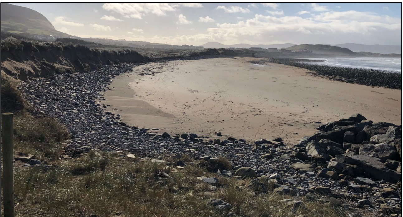
Figure 4.8: Extensive erosion south of the revetment at the WWTP, February 2022
