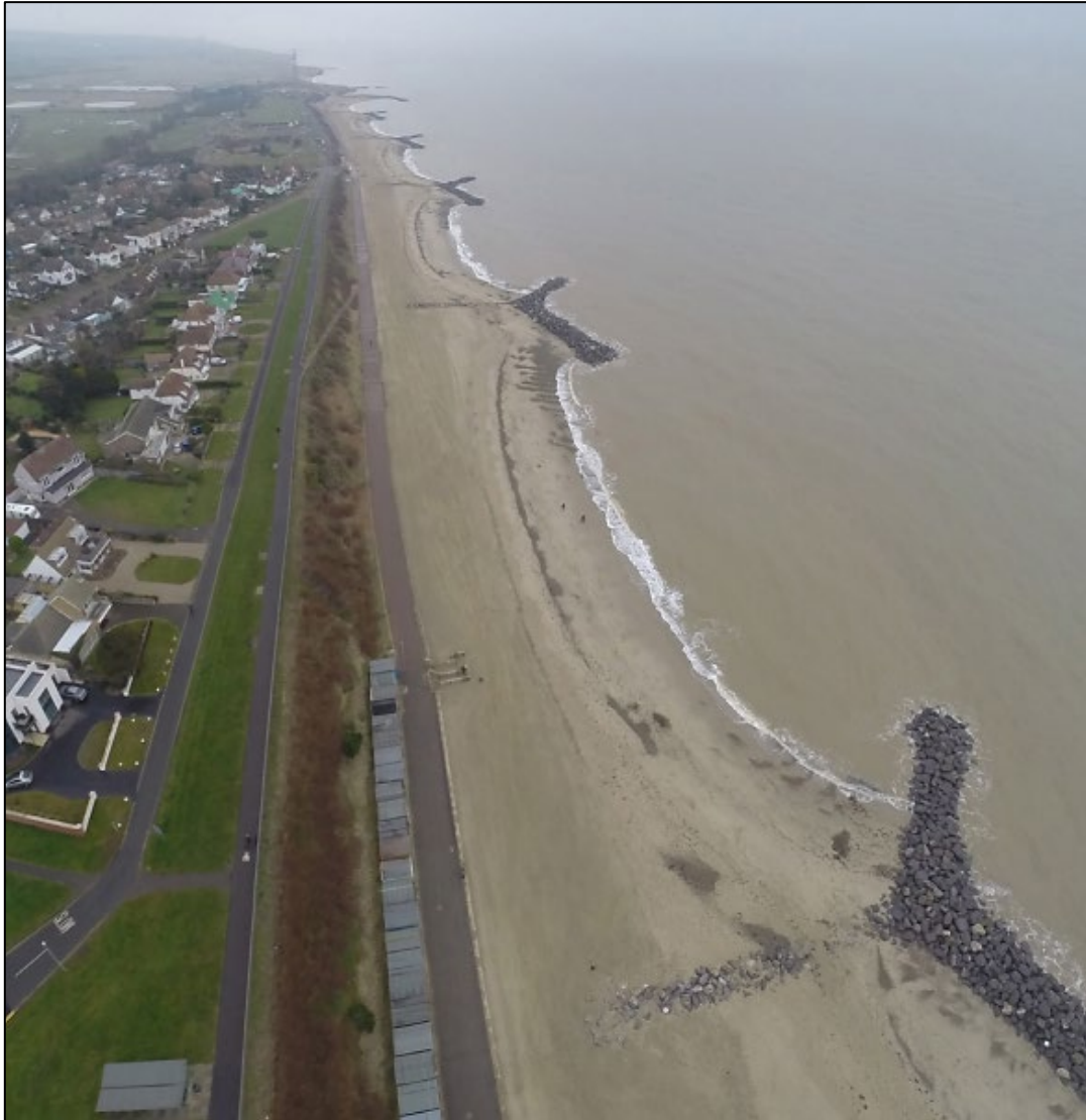
Figure 9.5: Aerial view of a fishtail groyne field at Clacton-on-Sea (VBACJV, 2019)
