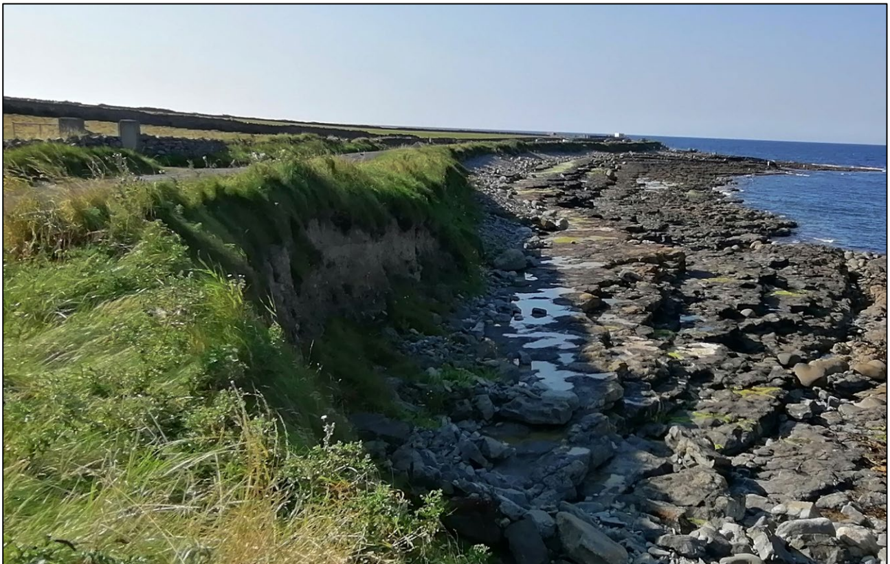
Figure 4.16: Evidence of localised wave-induced erosion at Easkey, Sept 2021
