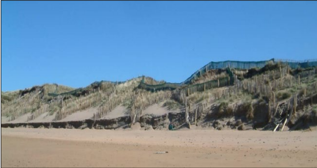
Figure 9.12: Sand trap fencing at a beach in Co. Clare
