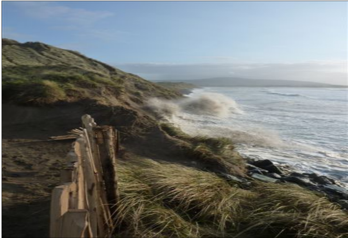
Figure 4.3: Damage to a considerable length of the dunes during large high tides on 11th May 2011
