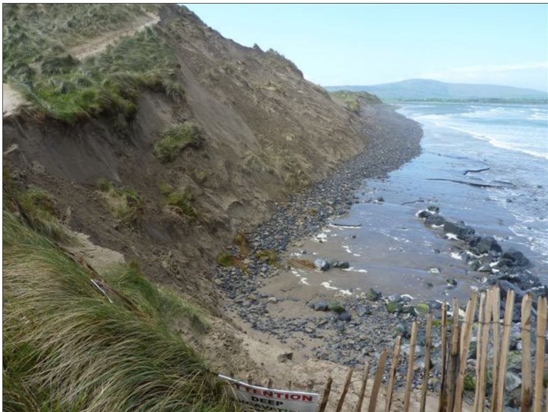
Figure 4.4: Resultant damage to the dunes south of Strandhill which also exposed a peat layer on 24 th May 2011.
