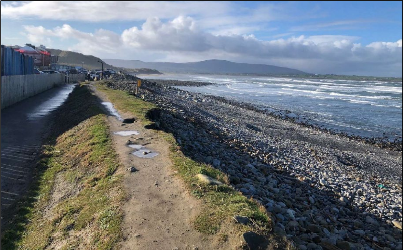
Figure 3.7: Example of cobble basement layer just north of Strandhill in February 2022
